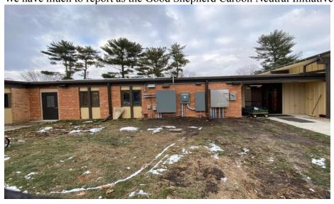
After a long delay due to supply chain issues, the new 600 amp service entrance was bored into the church from the relocated Alliant transformer. There are several large electrical boxes now installed on the south side of the Education Wing.
